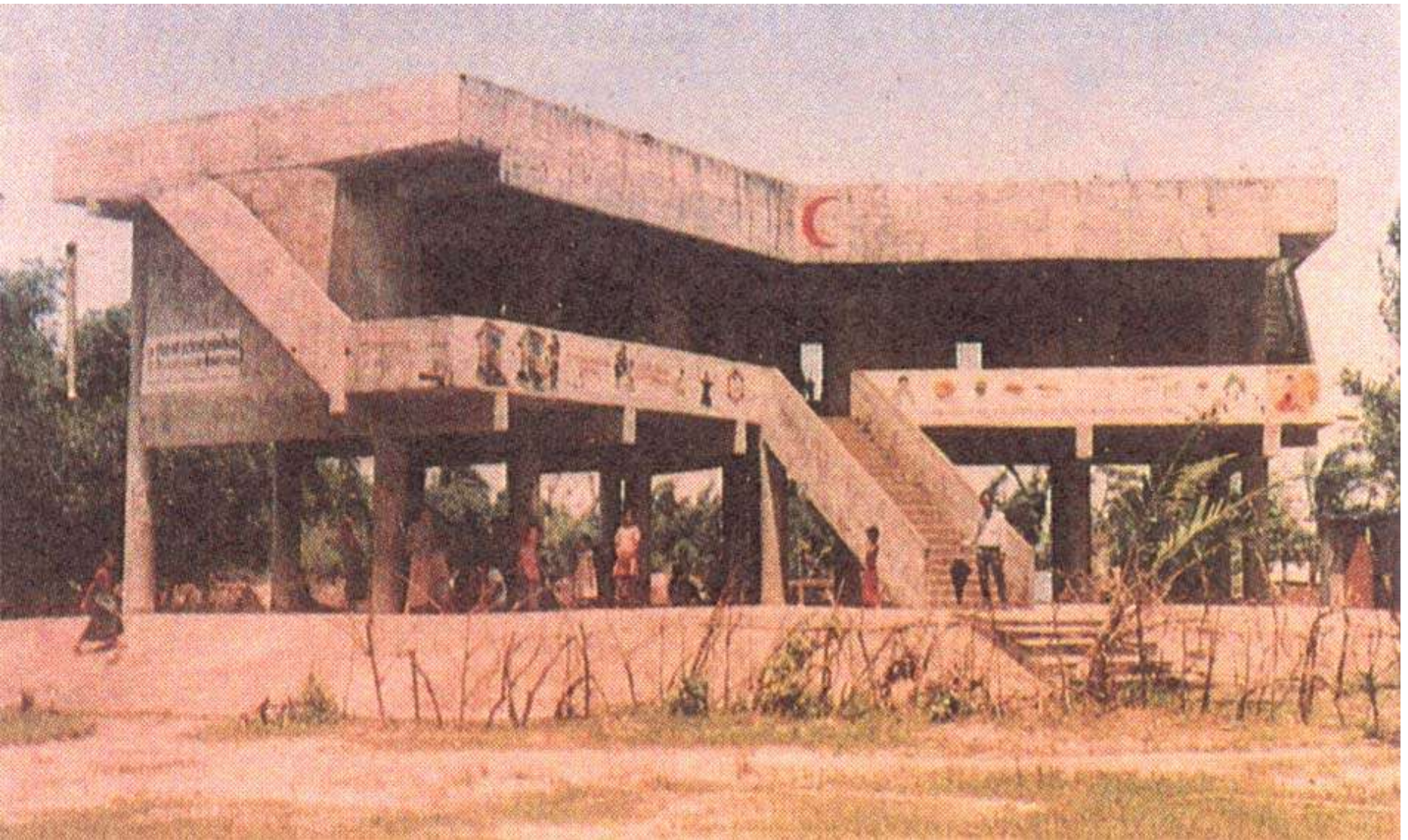
Multipurpose Cyclone and Storm Surge Shelter (Red Crescent Society)
