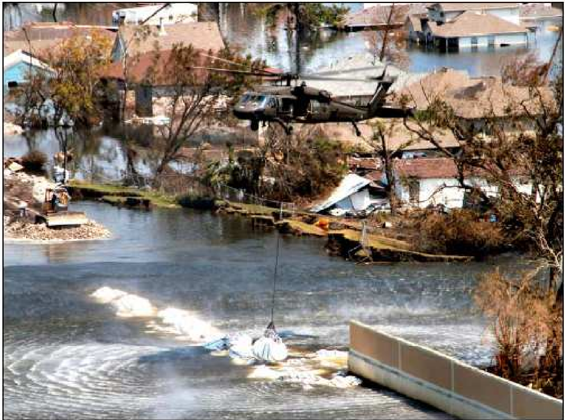
Levee Breach at the 17th Street Canal in New Orleans, LA – Photo: US Army Corps of Engineers (2005)
